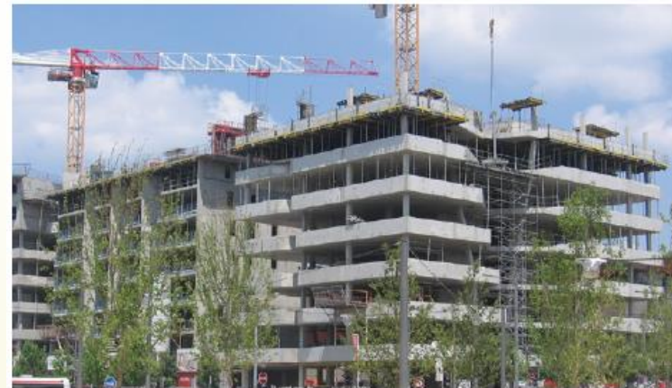
Core construction of the Hikari building in Lyon
