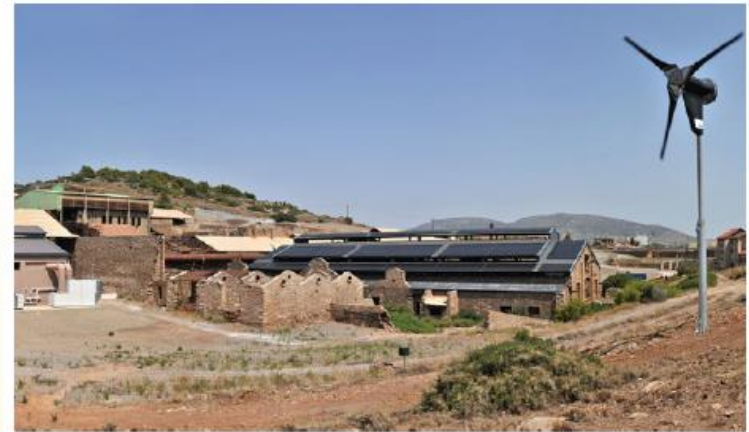
View of the Lavrion demo installation
