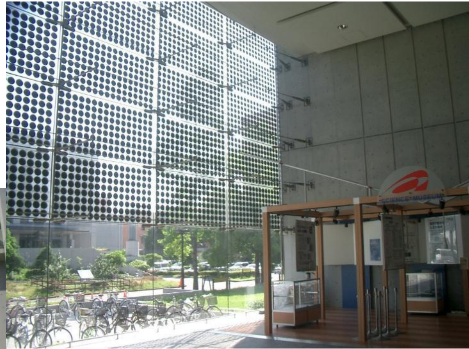
Tsukuba building, view from inside
