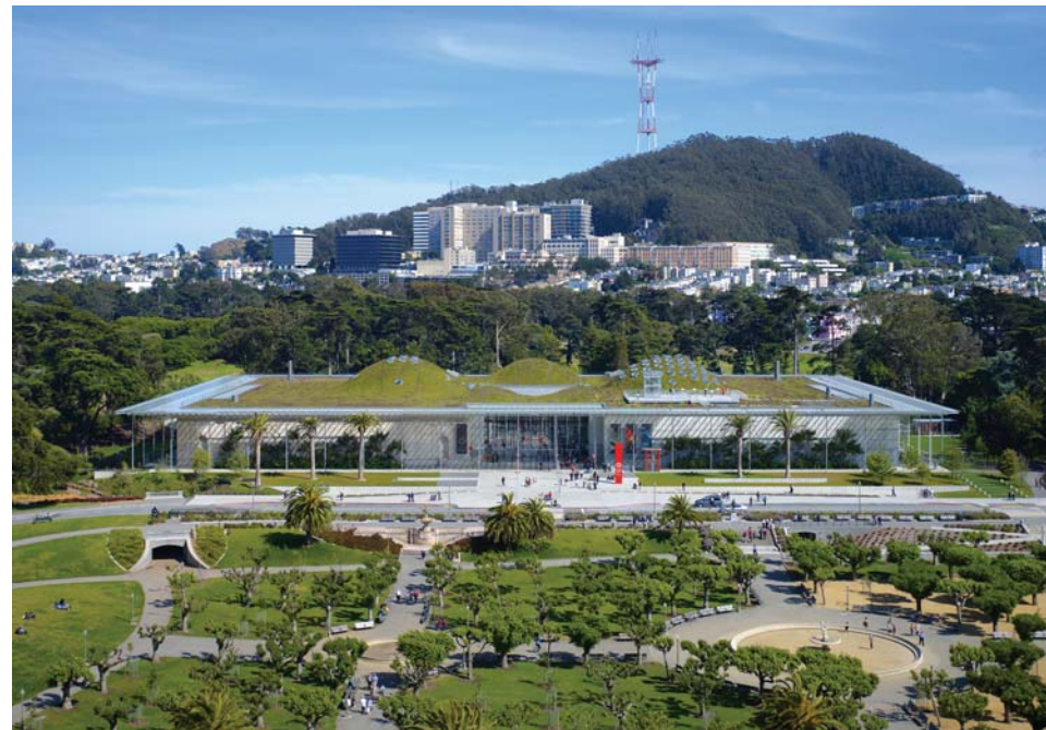
California Academy of Sciences Completed 2008 San Francisco, USA Renzo Piano Building Workshop BIPVs are applied on the canopy
