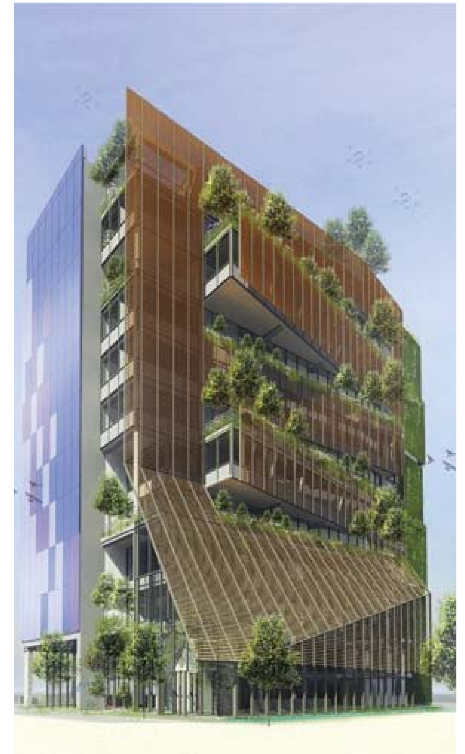
Ferrer Research & Development Center Design Development Barcelona, Spain William McDonough + Partners BIPVs are applied on the facade
