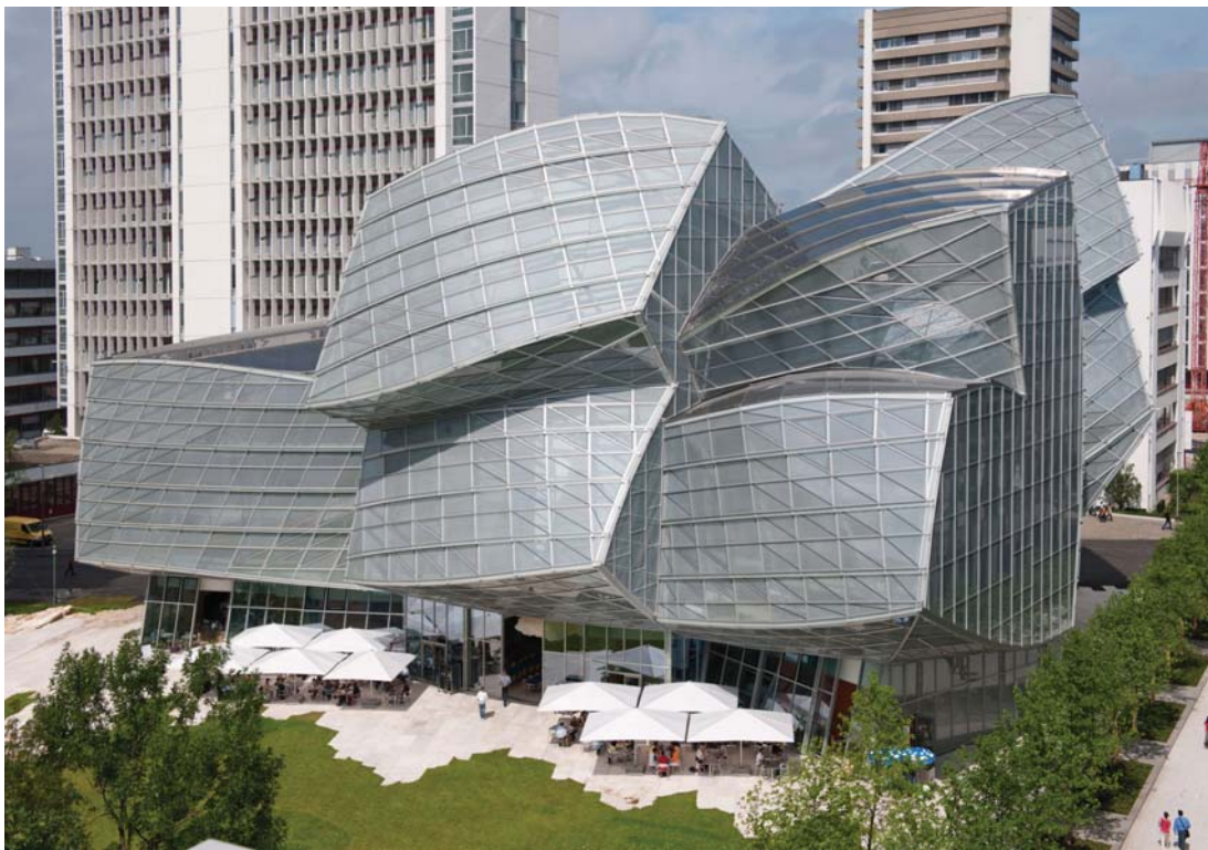
Novartis Basel Campus Completed 2009 Basel, Switzerland Gehry Partners BIPVs are applied on the roof
