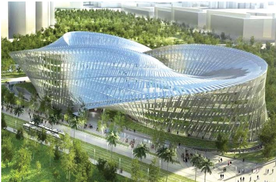
Taichung City Cultural Center , Swallow's Nest Competition Entry Taichung, Taiwan Vincent Callebaut Architectures BIPVs are applied in the envelope
