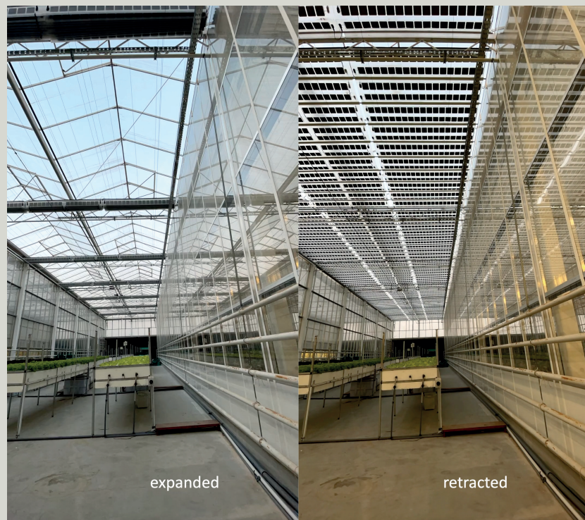
Figure 9: The Photovoltaic screens can be retracted and expanded
