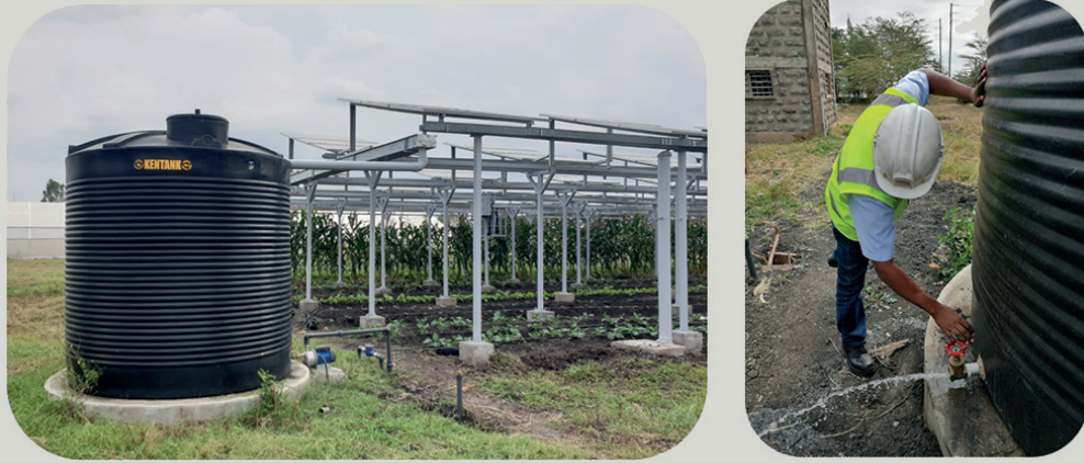
Figure 10: Proof of concept for the rainfall collection beside an Agri-PV system
